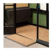
The low threshold (1.25 cm / 0.5 in) and the external platform makes it easy to access the pod with a wheelchair.
